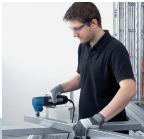
Cut-to-fit cable trays
