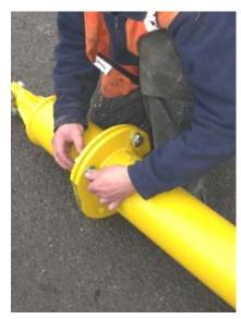
Lay out the beam struts end to end in the correct configuration, using the flats on each flange to prevent rolling. There are 3 x 2m beam struts on top of the stillage with a 1m strut and two end sections inside the stillage.
