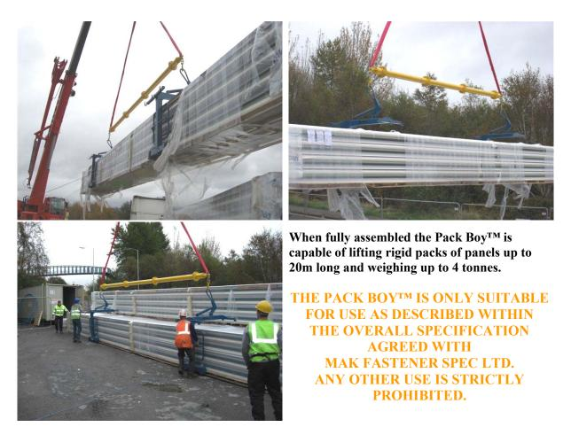
Once unloading is complete, the Pack Boy<sup>™</sup> must be carefully taken apart and returned to the storage stillage. All components must be secured in readiness for carrier collection.
