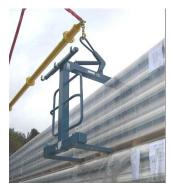
When positioning the Pack Boy<sup>TM</sup> in the panel pack, pay attention to load balance and ensure that the crane forks are fully inserted into the pack up to the heel of the forks. The use of push rods to aid insertion of the forks into each pack will avoid the need to climb on the delivery vehicle.
