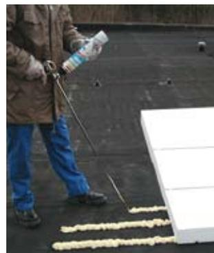
Extra long reaching polyurethane foam gun (1m in length), specially designed for roofing applications, in conjunction with Soudatherm Roof 250.
