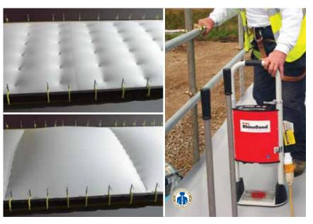
The RhinoBond welded membrane spreads the wind load evenly across the roof (top) as opposed to the traditional in-seam fixing method (bottom).
