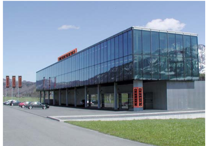
Leister Corporate Center in Kaegiswil, Switzerland.
