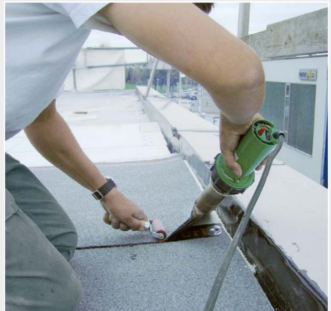
The powerful ELECTRON with a wide slot nozzle in use for welding bitumen.
