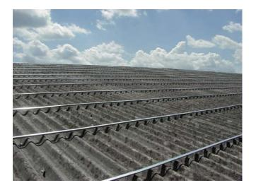
Gridtite installed over an old fibre cement roof prior to over cladding with steel sheets
