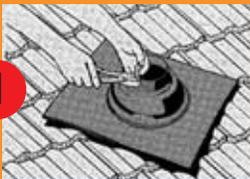
Trim Dektite® cone to suit pipe size using sharp tin snips.
