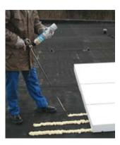
Extra long reaching polyurethane foam gun (1m in length), specially designed for roofing applications, in conjunction with Soudatherm Roof 250.
